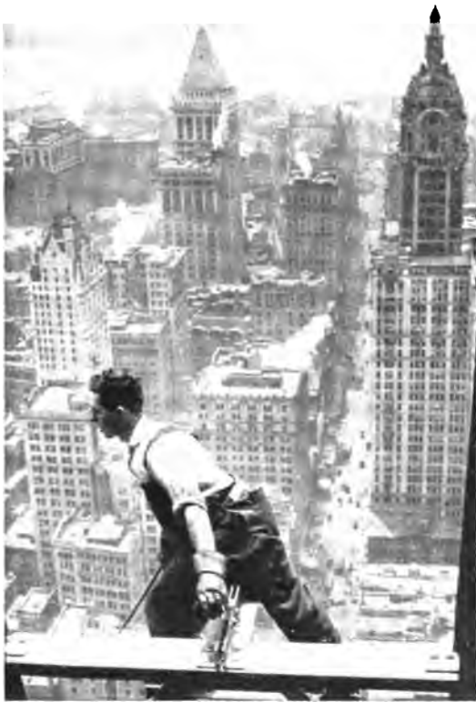
Photograph by Brown Brothers. THROWING A RED-HOT BOLT TO A RIVETER—FIVE HUNDRED FEET ABOVE THE PAVEMENT.
